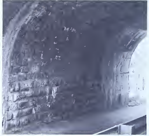
Reading Railroad bridge at Second and Hanover Streets, Hummelstown; one of the earliest stone railroad bridges built in the U.S. (1860); local limestone and "brownstone" were used.
